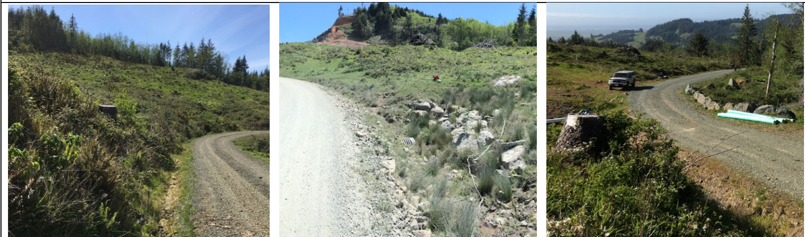
Photos 18A and 18B (left & center) – View W at main access road ditch. Photo 18C (right) – View NW at north access road ditch.
